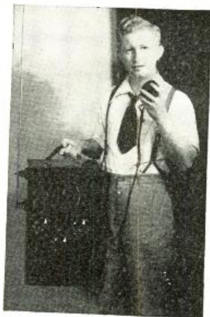
The portable 2½ meter A transceiver—it carries 2-way phone.
